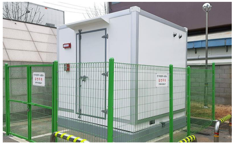
2024 Incheon City Building ESS (for peak reduction) - Incheon Integrated Business Center (300kWh)
