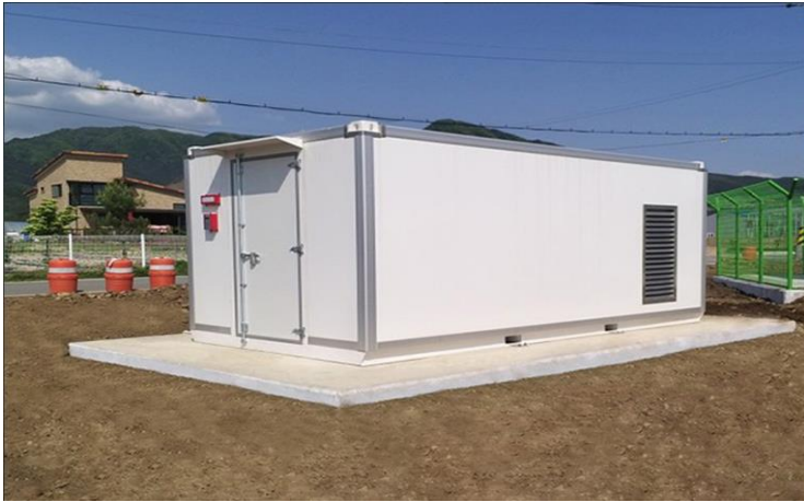
ESS for Gangwon-do buildings in 2021 (peak reduction) Gangwon-do Agricultural Research & Extension Services(250kWh)
