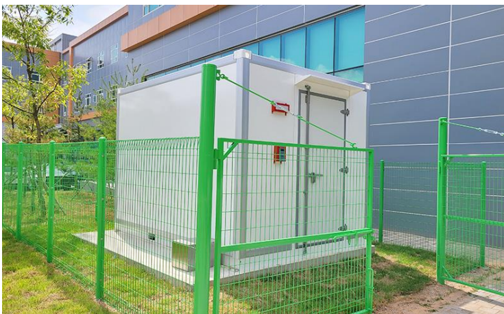
ESS for buildings in Iksan City in 2023 (peak reduction) - Korea Food Industry Cluster Promotion Agency (600kWh)
