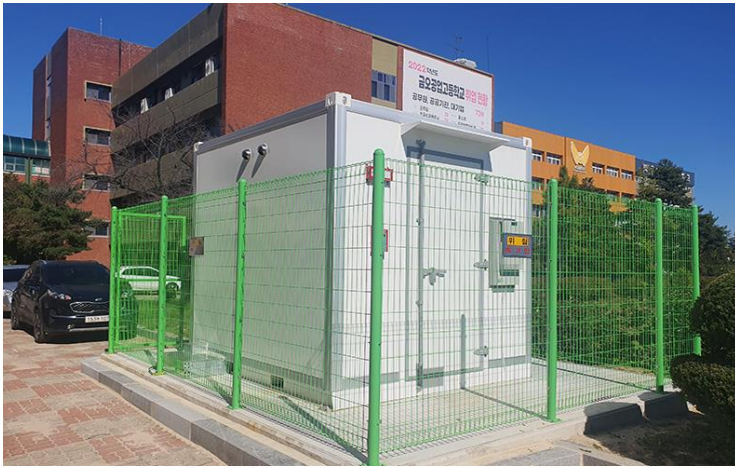
ESS for buildings in Gumi City in 2023 (for peak reduction) - Geumo Technical High School (150kWh)
